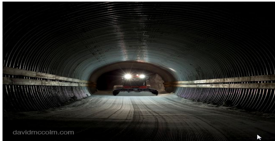
New Tunnel under the Women's Track!
